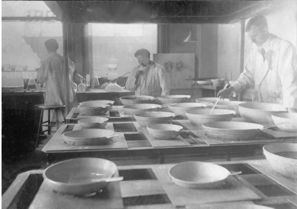
5.6 The fractional crystallization laboratory was in the northeast corner of the 5th floor. Over each burner is an asbestos sheet with a circular cutout to hold the round-bottomed porcelain bowls containing the radium-barium salt solutions. Overhead is a hood to vent the steam and acid fumes. The progression of the process is reflected in bowl sizes – the salts in the smaller bowls contain richer concentrations of radium. Photo c.1915. On the right is Glenn D. Kammer. ORAU
