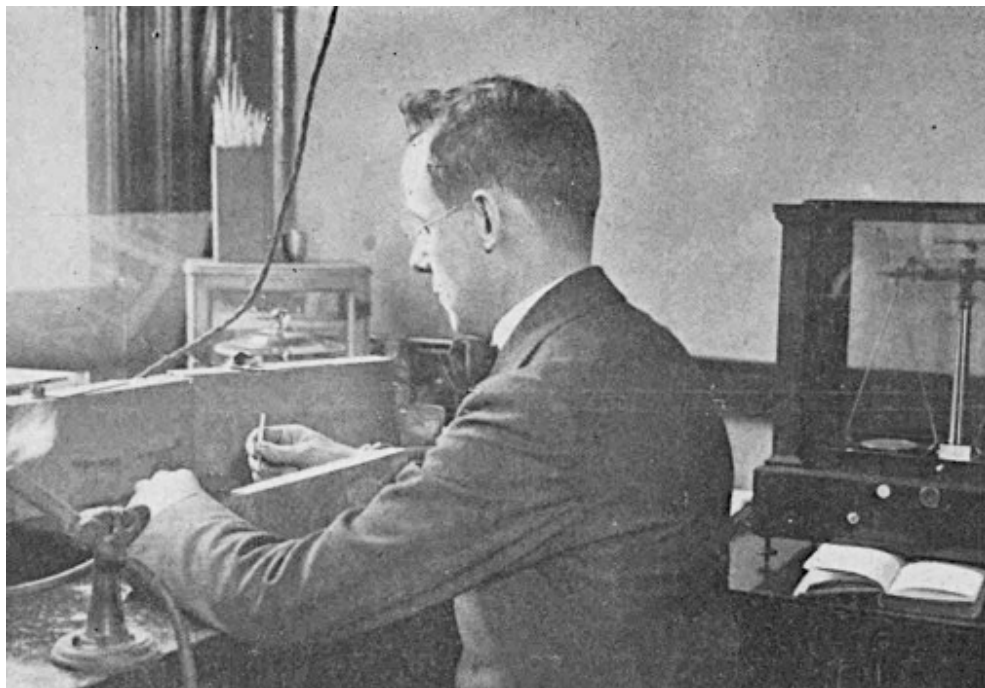
5.10 Left, Glenn D. Kammer tubing Marie Curie's radium, c. 1921. There are no contamination controls. A lead "shadow" shield in the front is a recent addition to reduce radiation exposure of his torso. CPP
