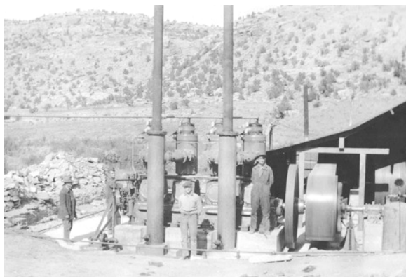
3.27 Left, the Fairbanks-Morse diesel engines to power the generators are up and running. Later, the engines were enclosed in a building. RHS 3.28 Right, SCC reserved a fleet of narrow-gauge railroad tank cars to deliver the diesel oil to Placerville. From Placerville, trucks hauled the oil to the Joe Jr. site. RHS
