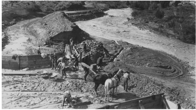
3.21 Left, construction of the Joe Jr. mill in 1914 included digging a ditch to divert San Miguel River water to the mill powerhouse. HHC4 3.22 Right, a view of the ditch looking downstream. In the foreground is the short spillway to carry Hieroglyphic Canyon storm water over the ditch. The San Miguel River is on the right and the horses face the direction of the flow of the canyon drainage. HHC4
