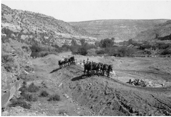
3.21 Left, construction of the Joe Jr. mill in 1914 included digging a ditch to divert San Miguel River water to the mill powerhouse. HHC4 3.22 Right, a view of the ditch looking downstream. In the foreground is the short spillway to carry Hieroglyphic Canyon storm water over the ditch. The San Miguel River is on the right and the horses face the direction of the flow of the canyon drainage. HHC4
