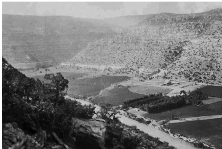
3.16 An early photograph of the SCC Joe Jr. mill site (and later Uravan). The view is looking south across the San Miguel River toward the end of Hieroglyphic Canyon — the notch in the hillside left of center in the upper half of the picture. The mill complex was built on the flatland between the canyon notch and the ranch on the right. ORAU
