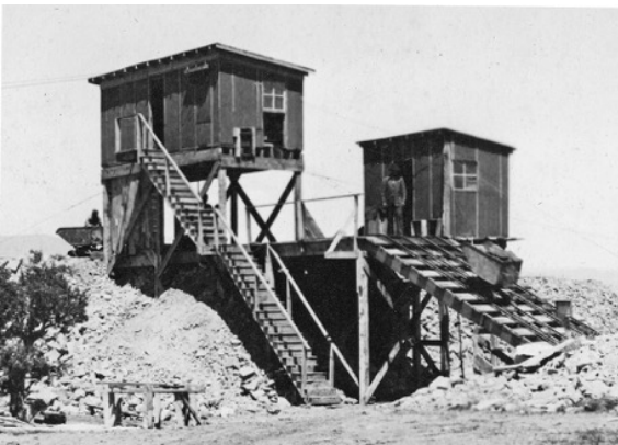
3.11 Left, headhouse of the inclined mine shaft #2 at Club Camp. An ore car is on the incline; another is at the rear being unloaded. HHC4 3.12 Right, the ore was sorted inside the tent. Ore destined for the mill went to the ore bin on the right for loading into wagons. Higher-grade ore was separated and bagged for shipment to the Placerville railhead. Waste rock was discarded to the sides. HHC4
