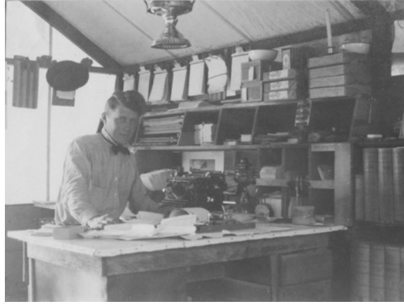
3.32 John Galley at work. RHS
